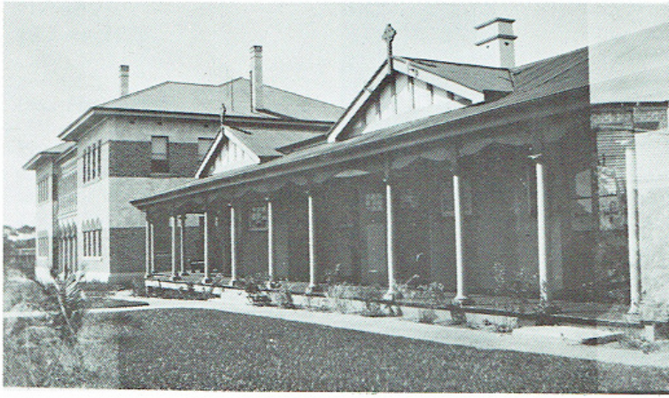
Building in foreground second convent formerly Brockhurst Hospital 1928
