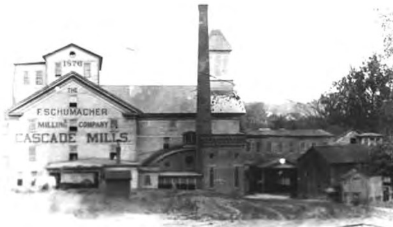
Ferdinand Schumacher's Cascade Mill, Akron, Ohio circa 1878. Source: Cascade Locks Park Association.
